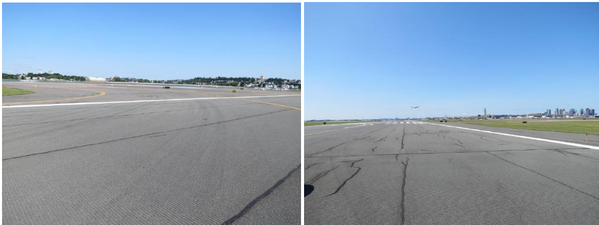
Figure 22. StellarFlex Fuel Resistant at Boston Logan International Airport Runway 4L-22R in 2014 after Ten Years of Service (Left) and a Federal Aviation Administration Item P-401 Mix in 2014 After Ten Years of Service at Boston Logan International Airport Runway (Right).
