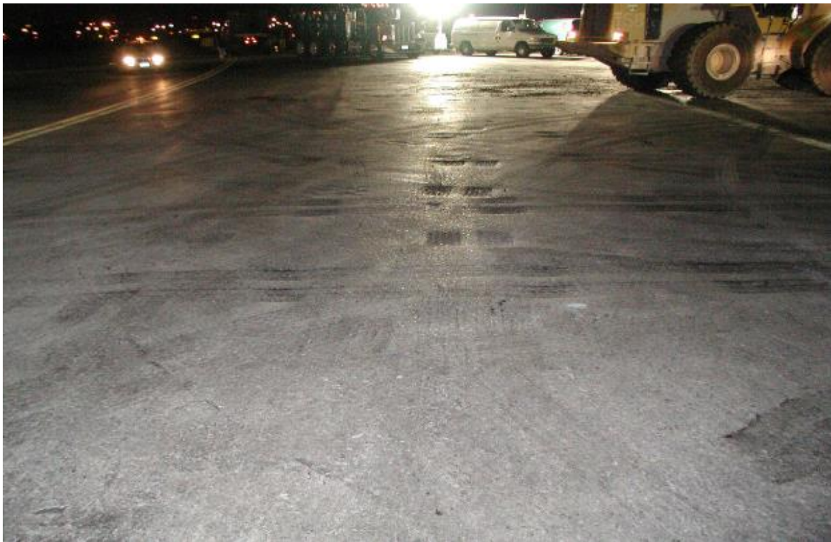
Figure 1. Depressions in Asphalt Surface Due to Fuel Spill Softening
