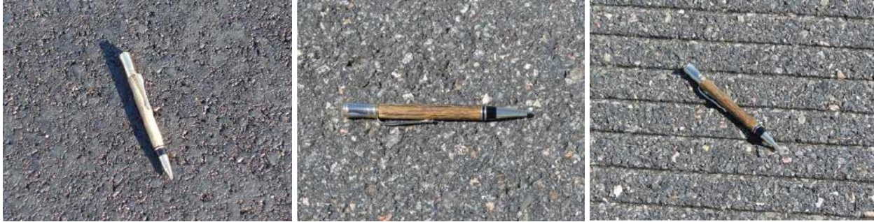
Figure 21. StellarFlex Fuel Resistant Texture at Boston Logan International Airport in 2004 (Left) and the Same Texture in 2014 (Middle and Right).
