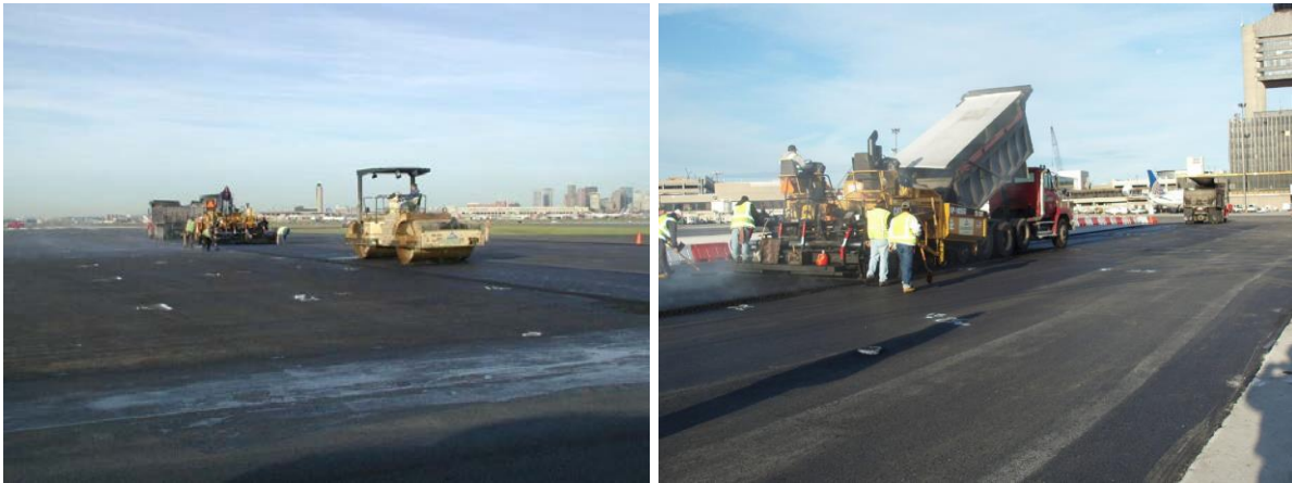
Figure 20. Placement of StellarFlex Fuel-Resistant (FR) on Boston Logan International Airport Runway 4L-22R (Left) and Alleyway B-C (Right)
