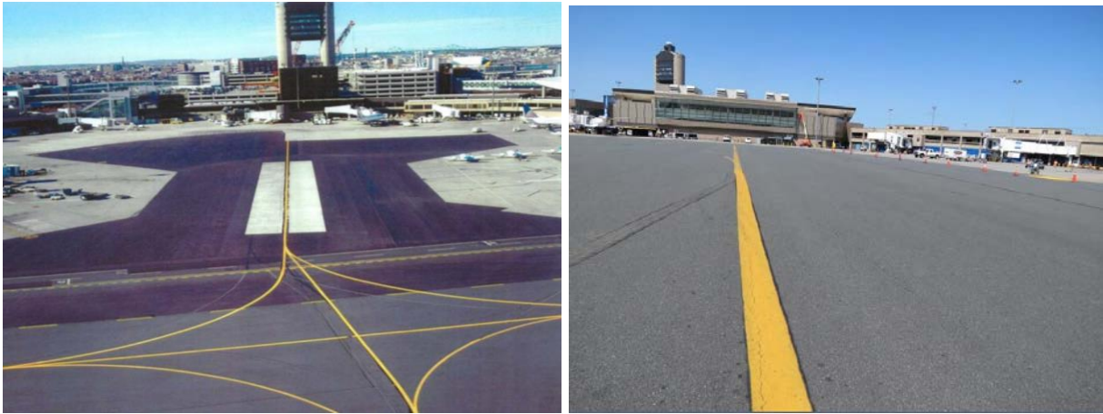
Figure 23. Newly Paved StellarFlex Fuel Resistant (FR) at Boston Logan International Airport Alleyway B-C in 2005 (Left) [17] and after 12 Years of Service (Right)
